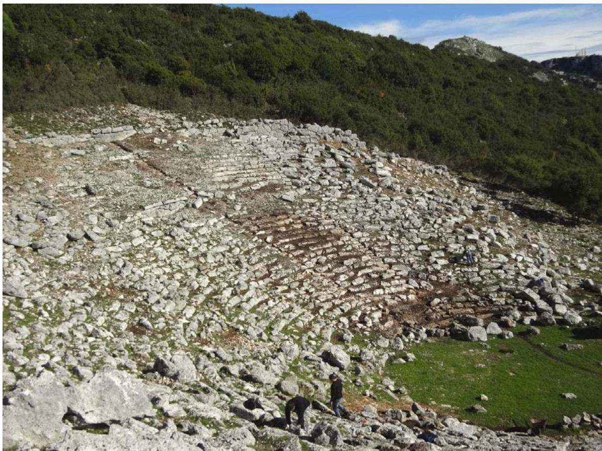
7. Revealing raw lines and preserved seats during the deforestation works. (photo: Diazoma/2012)
